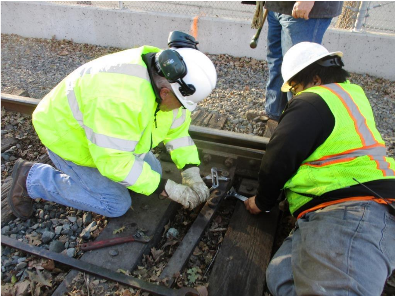
Bill and Anthony make adjustments to the position of the connecting rod on Switch 101
