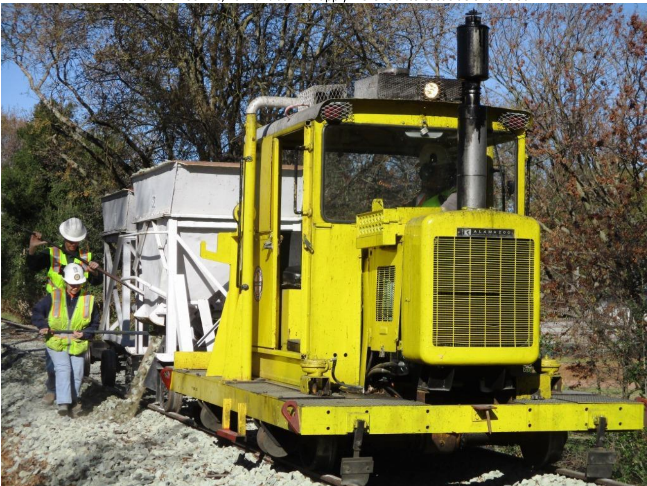
Steve keeps the Kalamazoo rolling slowly south as John C. and Pam discharge rock on the west rail
