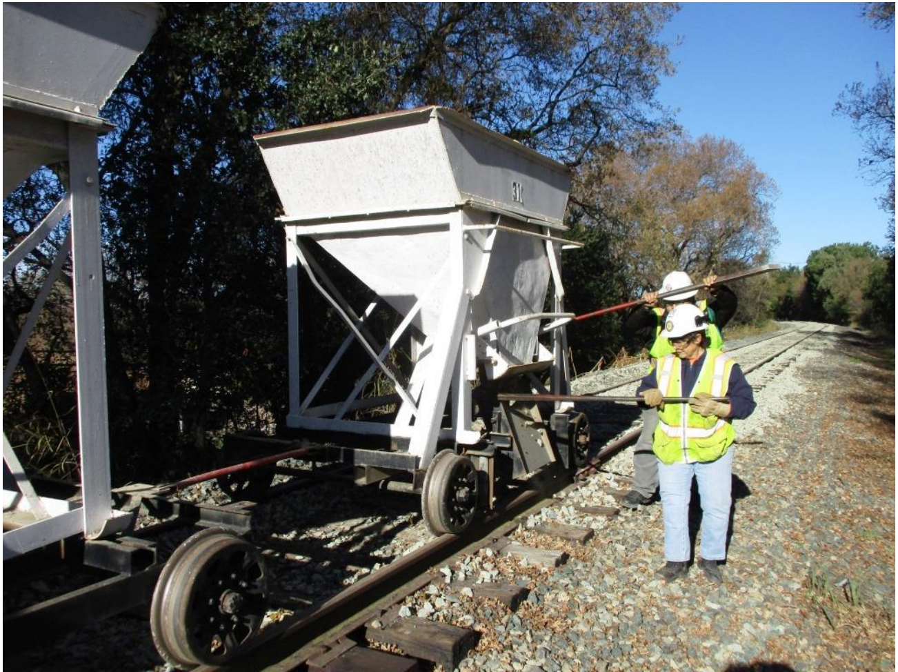
Pam and Anthony continue dropping rock further down the hill
