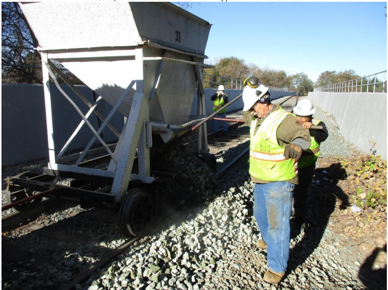
Clem and Anthony discharge rock from a side-dump hopper at the transition point between the I-5 Bridge and solid ground
