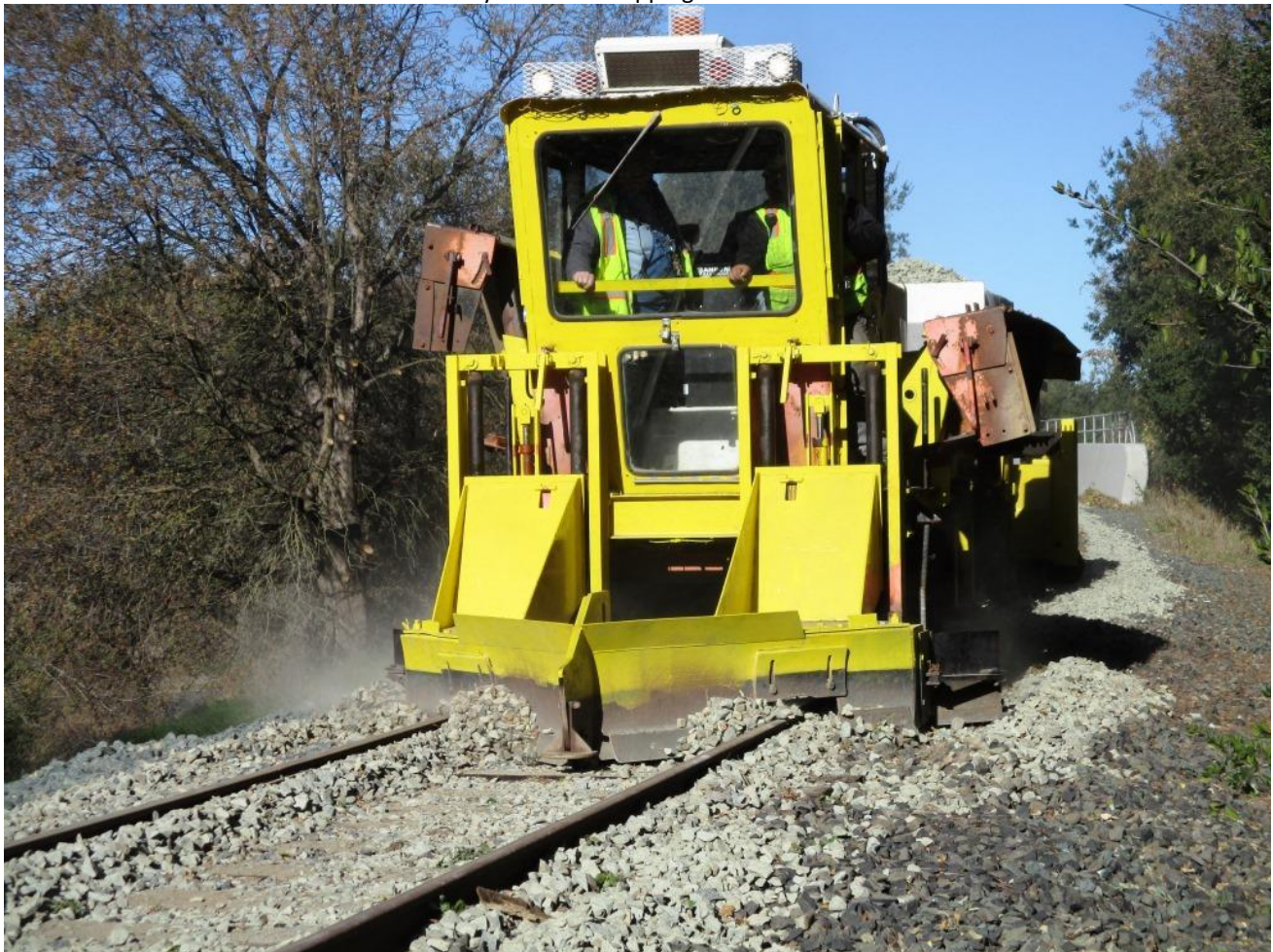
Chris C. brings in the ballast regulator with the plow down to spread the rock about the track
