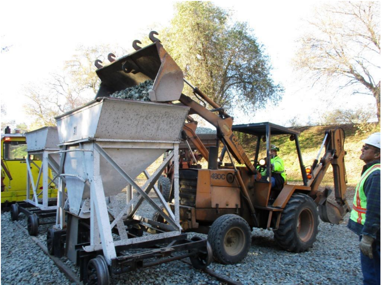
At Setzer, Mike F. in the back-hoe fills a hopper car with ballast-rock
