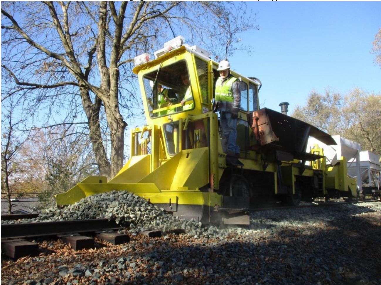
Mike M. keeps a close eye on the action as Chris C. in the regulator spreads the rock evenly about the track
