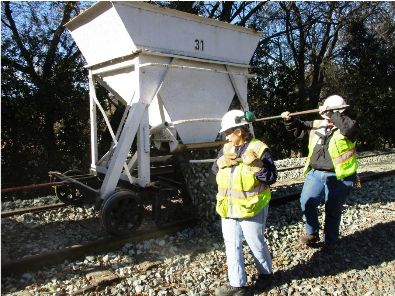
With another load of rock on site, Pam and Heather disgorge it onto the west side of the rail
