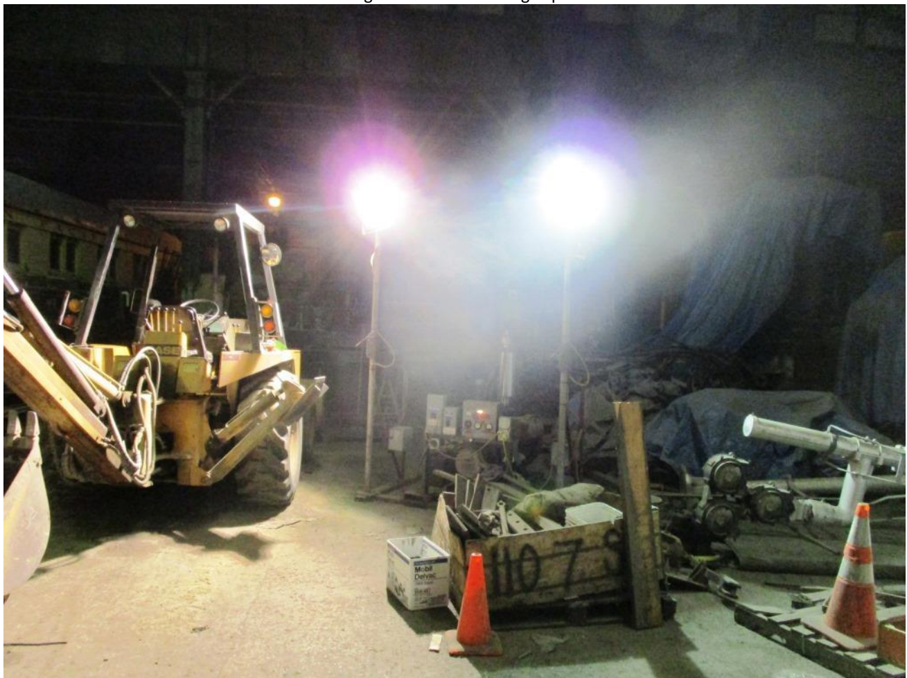
Fixed by Chris C., the MOW Team's light plant now puts out more lumens than Alpha Canis Majoris, the brightest star in the night sky
