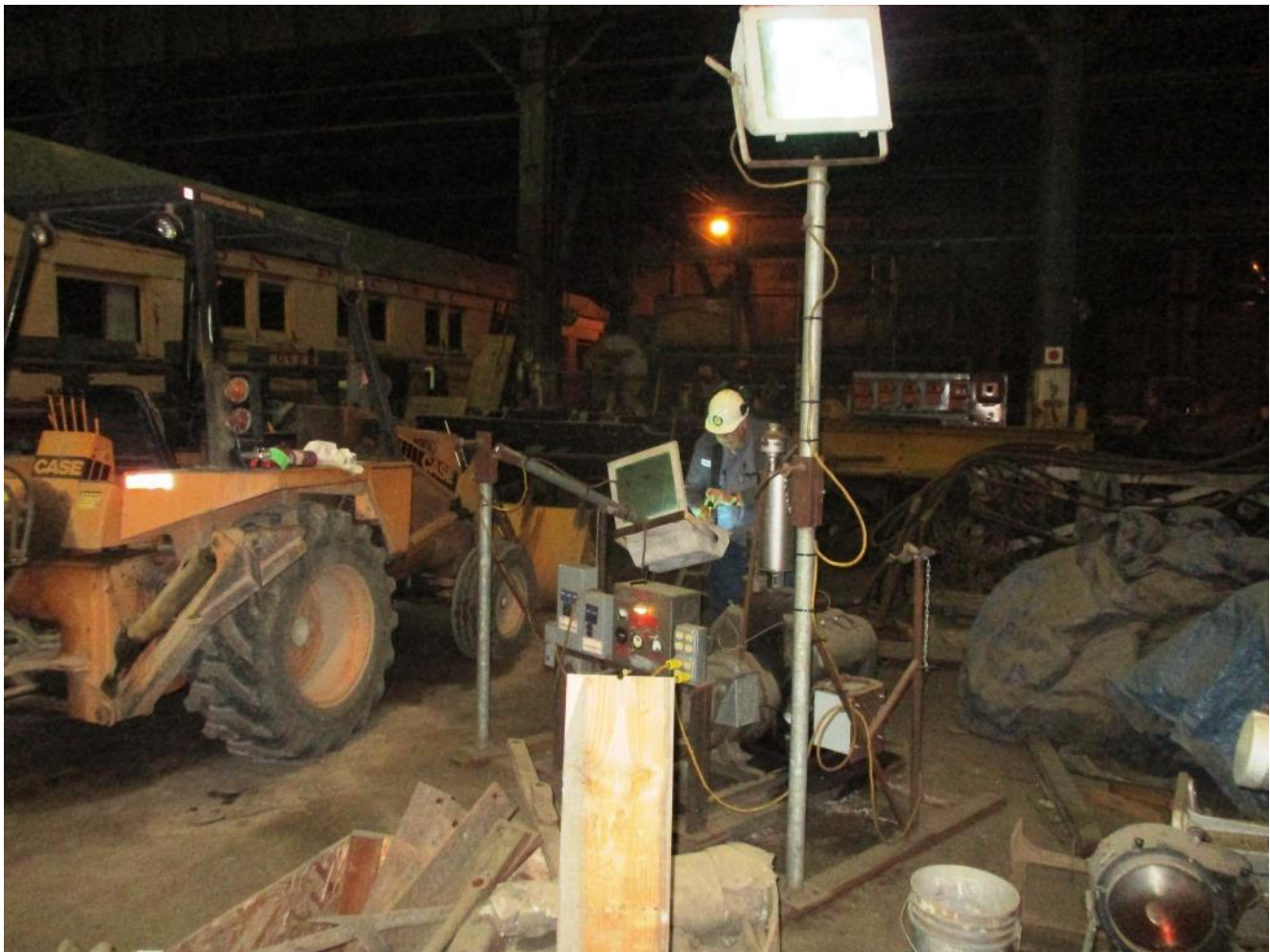
Chris C. returning the MOW Team's light-plant to service
