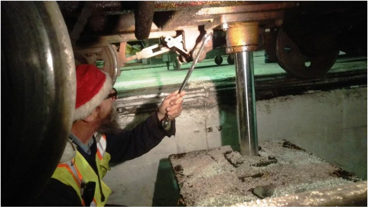
Joe, under the 125, finds the wonky hydraulic cylinder on its turntable and begins the process of removal
