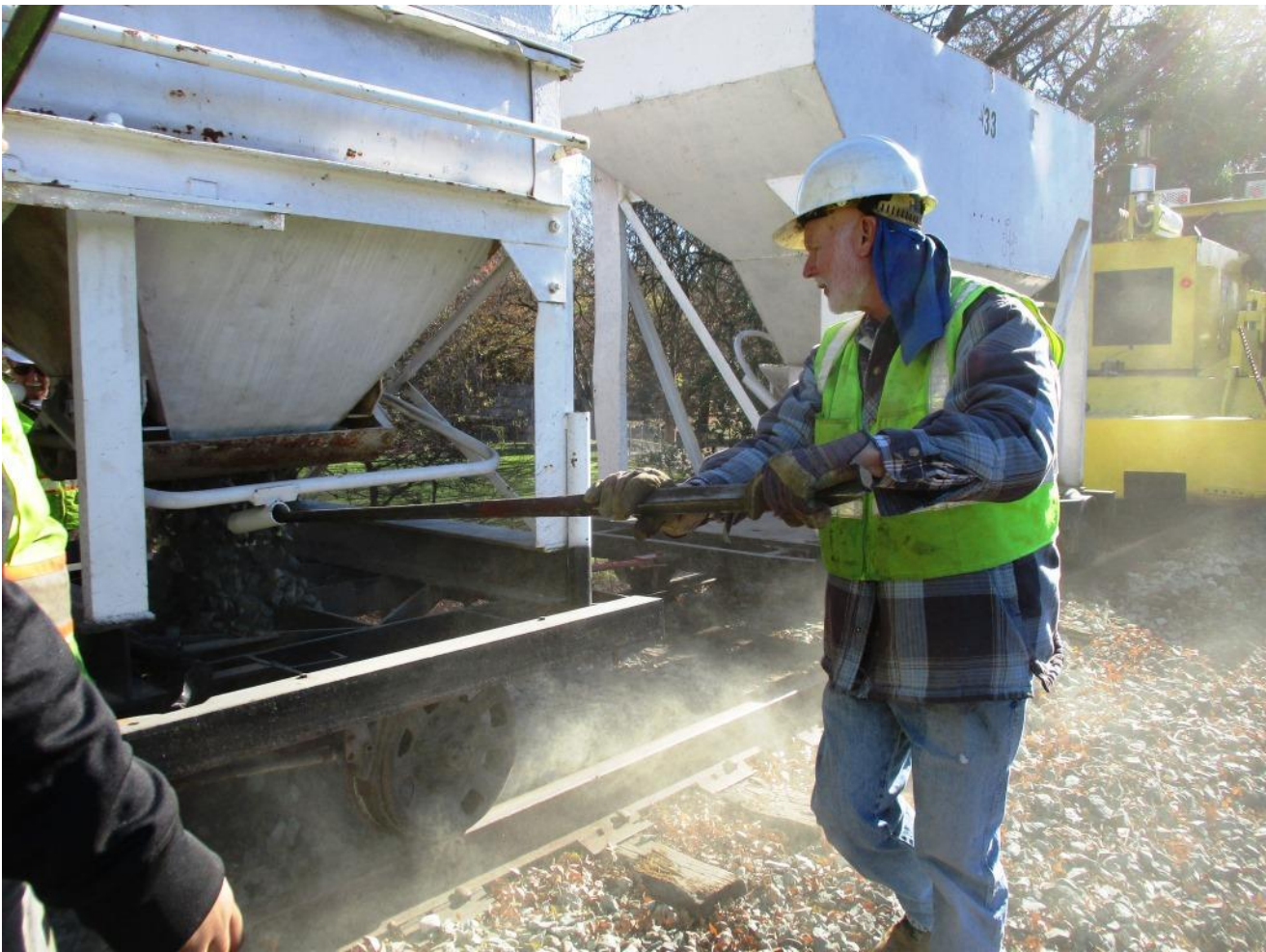
Mike M. disgorges rock from one of the center-dump hoppers
