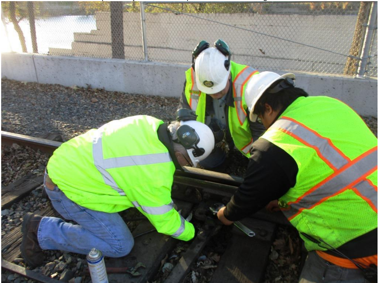
Chris C. inspects the new position of the connecting rod on the transit clip to see if the adjustment did the trick
