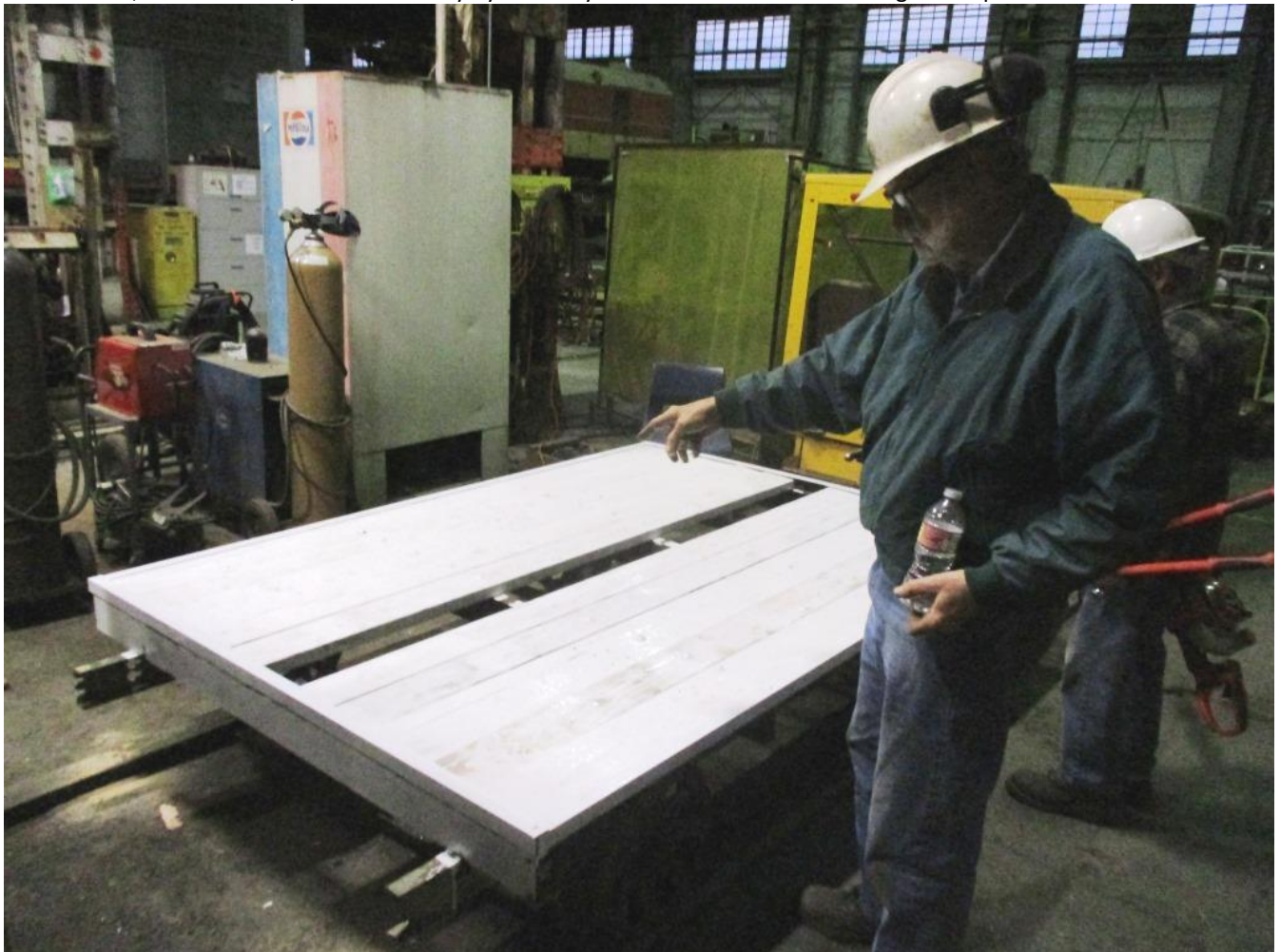
Alan describes how this flatcar that he's been building will accommodate the hydraulic power units and tools
